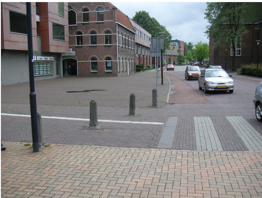
Figure 4: Torenstraat intersection approach with pedestrian crossing and cycle lane,
