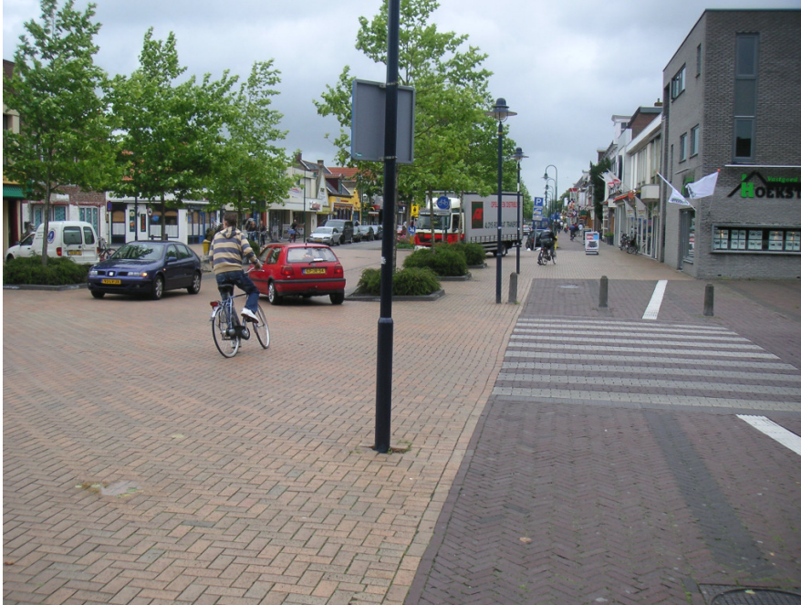
Figure 3: Noordkade/Zuidkade intersection approach with bollards for channelisation, Drachten, the Netherlands
